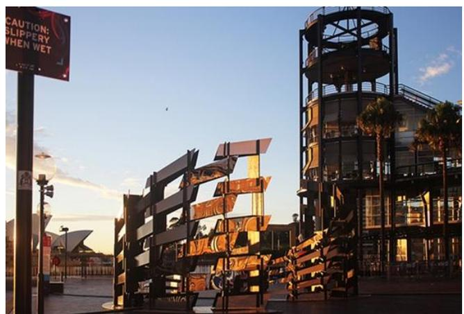
Figure 8: Ptolemi a reciprocal frame structure is made of timber and mirrored steel. Sydney 2016.
